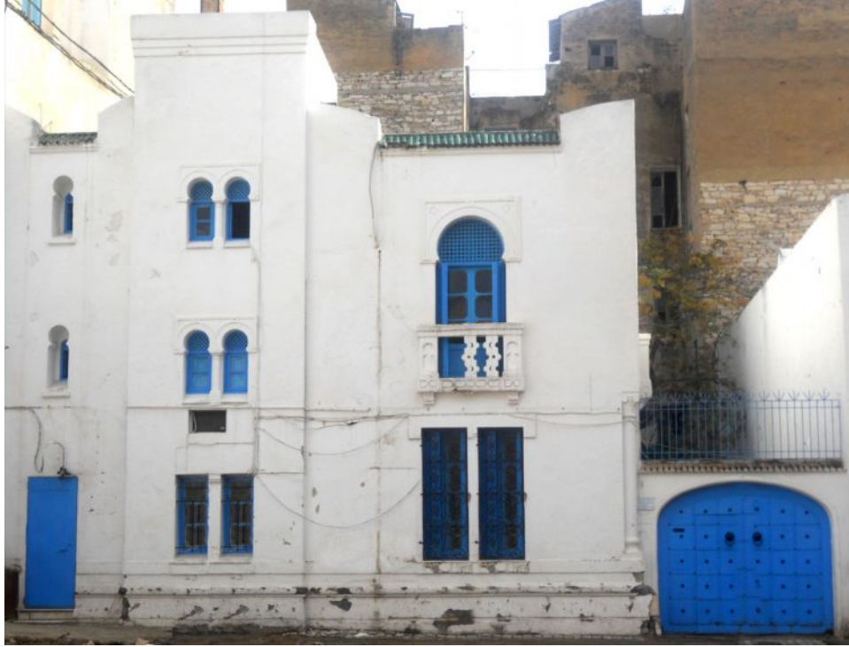
CEMAT villa "Maria Carlotta" seen in full for the first time due to construction next door.
